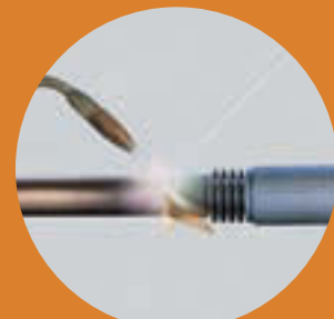
3 start brazing around the whole circumference saldare la circonferenza
